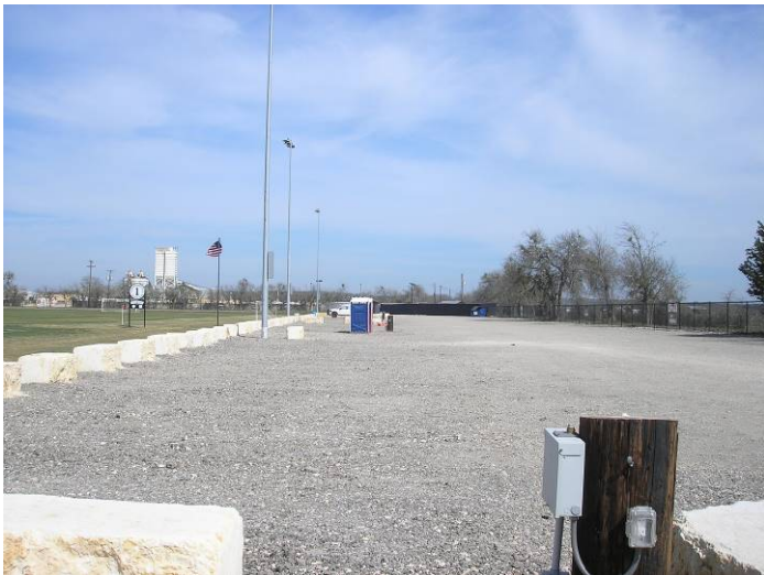
Photo #27 – View of the area immediately north of PRF #S-8.
