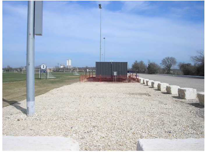
Photo #22 – View of the area immediately north of PRF #S-7.
