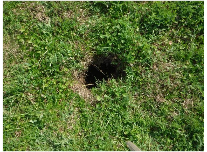
Photo #18 – View of PRF #S-5 observed in the south-central portion of the project site.
